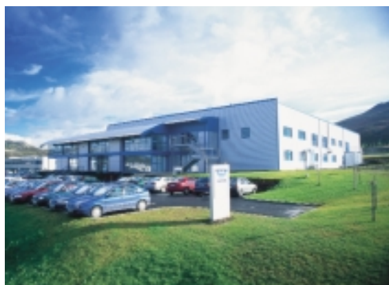
The Trinity Biotech facility at Bray, County Wicklow, Ireland
