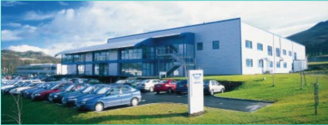
Corporate Headquarters, Dublin, Ireland.
